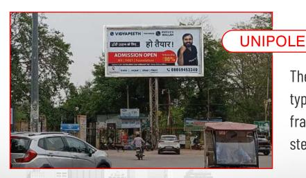
The Uni-pole is a large-format billboard type placed atop a very high pole. frame structure mounted atop a single steel pole or column.
